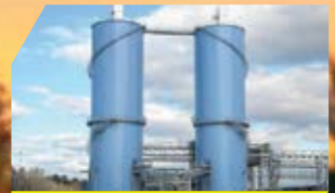
Dry Storage Tanks
